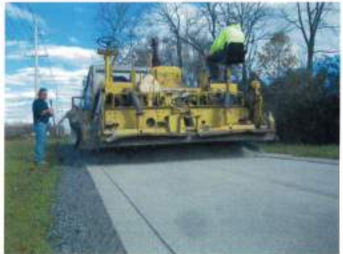
Paving a portion of the Phase One section
