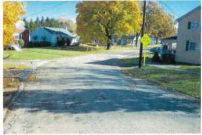
North Fairfield Street at Bunger Street looking north
