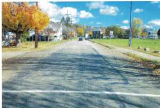
North Walnut Street near North Vincent Street looking north
