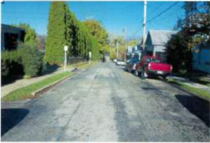
East Loyalhanna Street at Marker Street looking west
