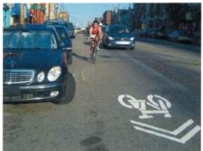
An example of an on-road route designated with a shared lane pavement marking, or sharrow (see page 64)
