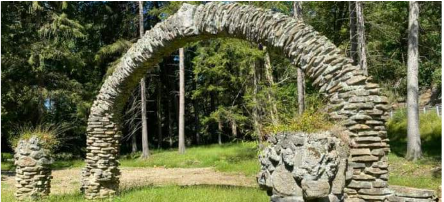
EXISTING HISTORIC STONE ARCHWAY
