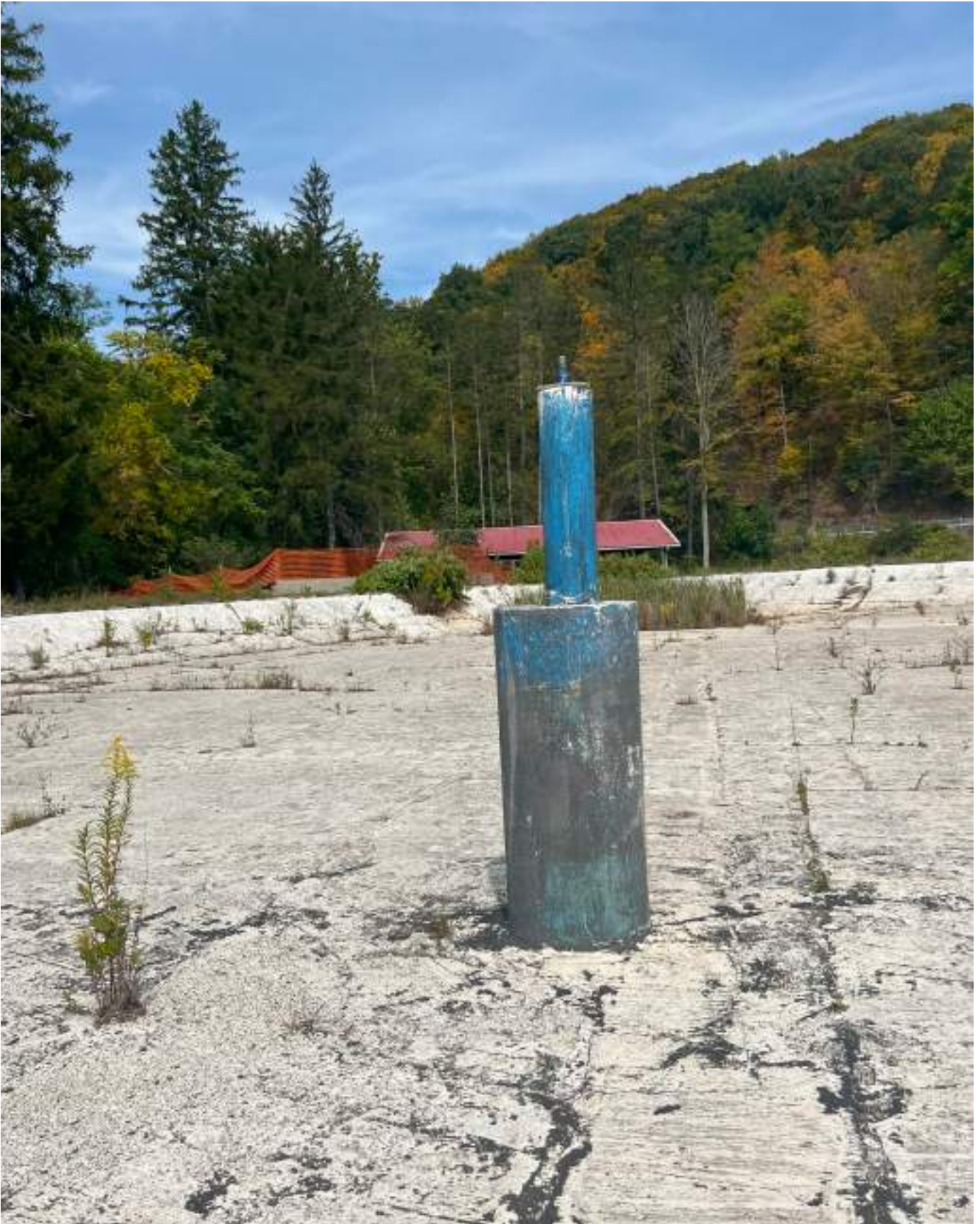
EXISTING POOL SHELL CONDITIONS
