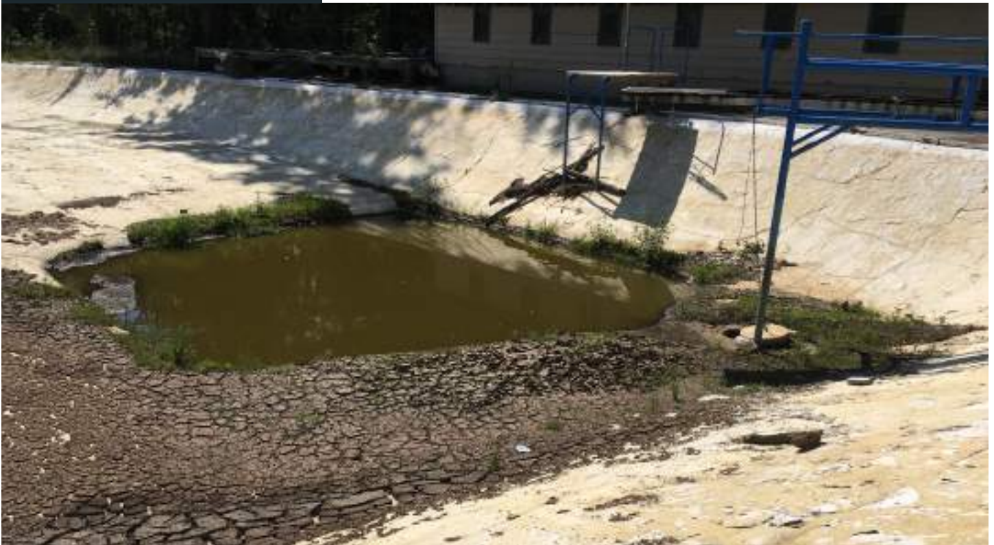
EXISTING POOL SHELL CONDITIONS
