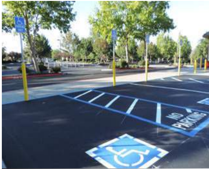
ADA PARKING WITH FLUSH CURBS
