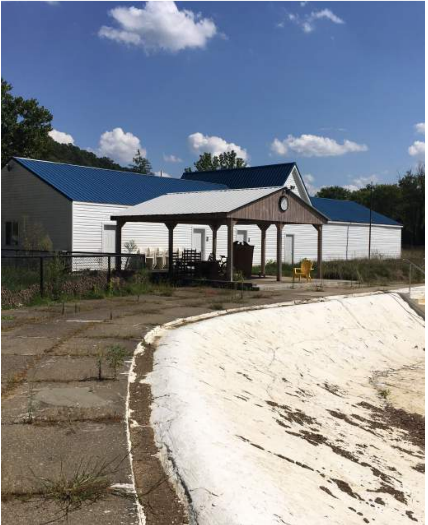
EXISTING POOL SHELL
