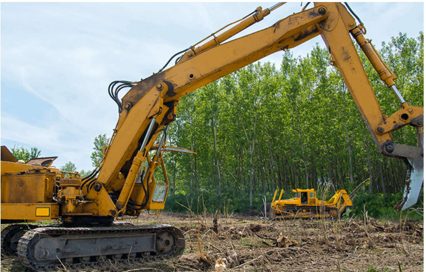
SITE CLEARING & GRUBBING
