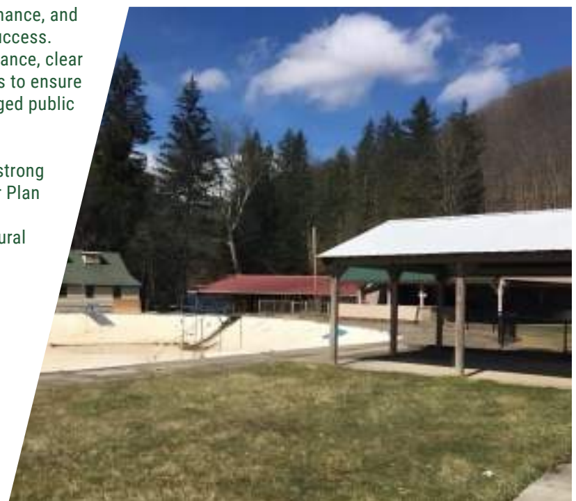
EXISTING SITE BEFORE BUILDING DEMOLITION
